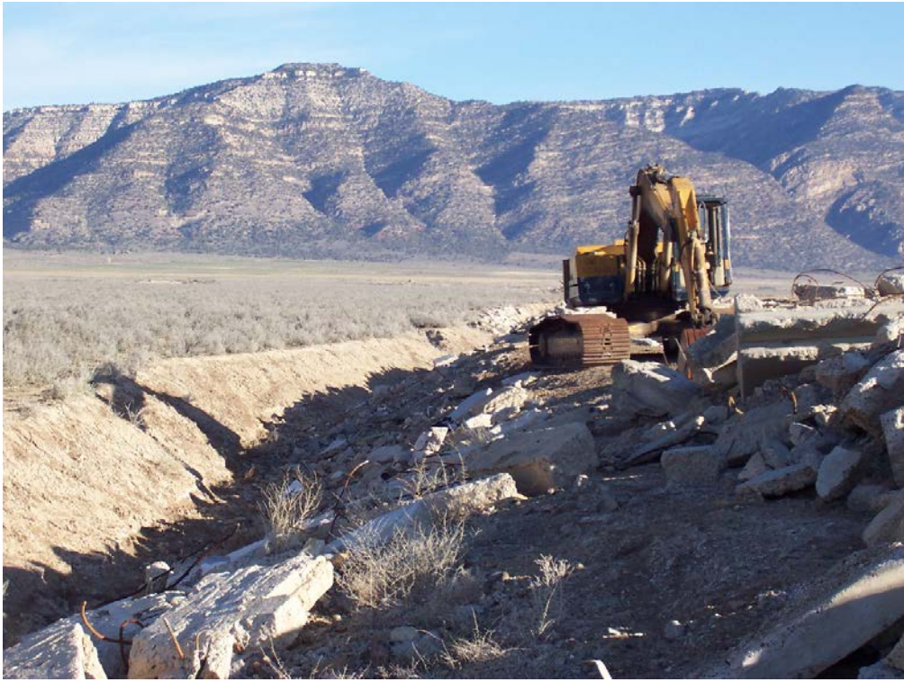
Equipment with concrete rip-rap on east side of channel
