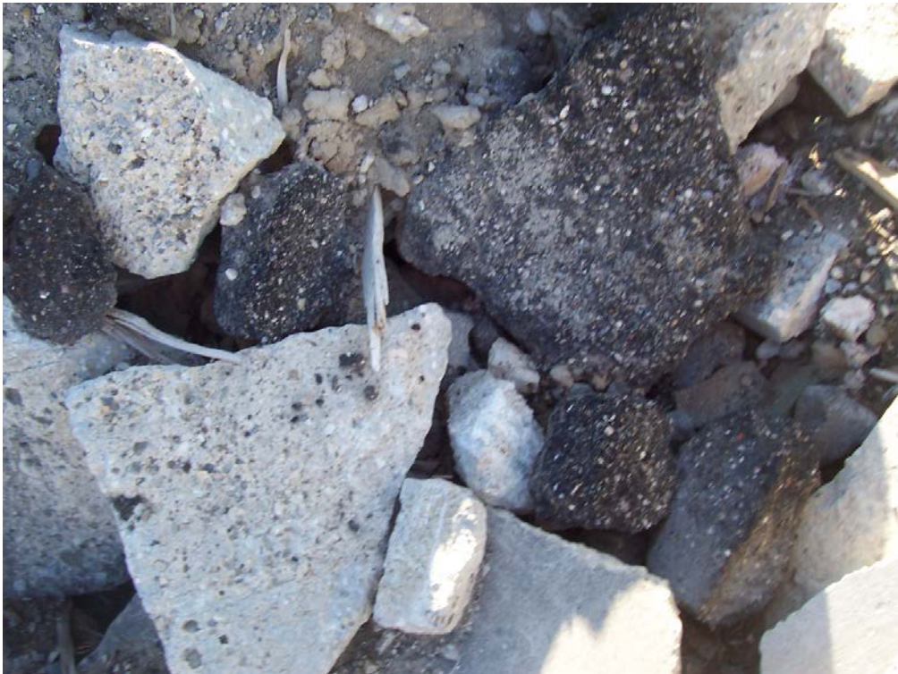
Close up of asphalt debris
