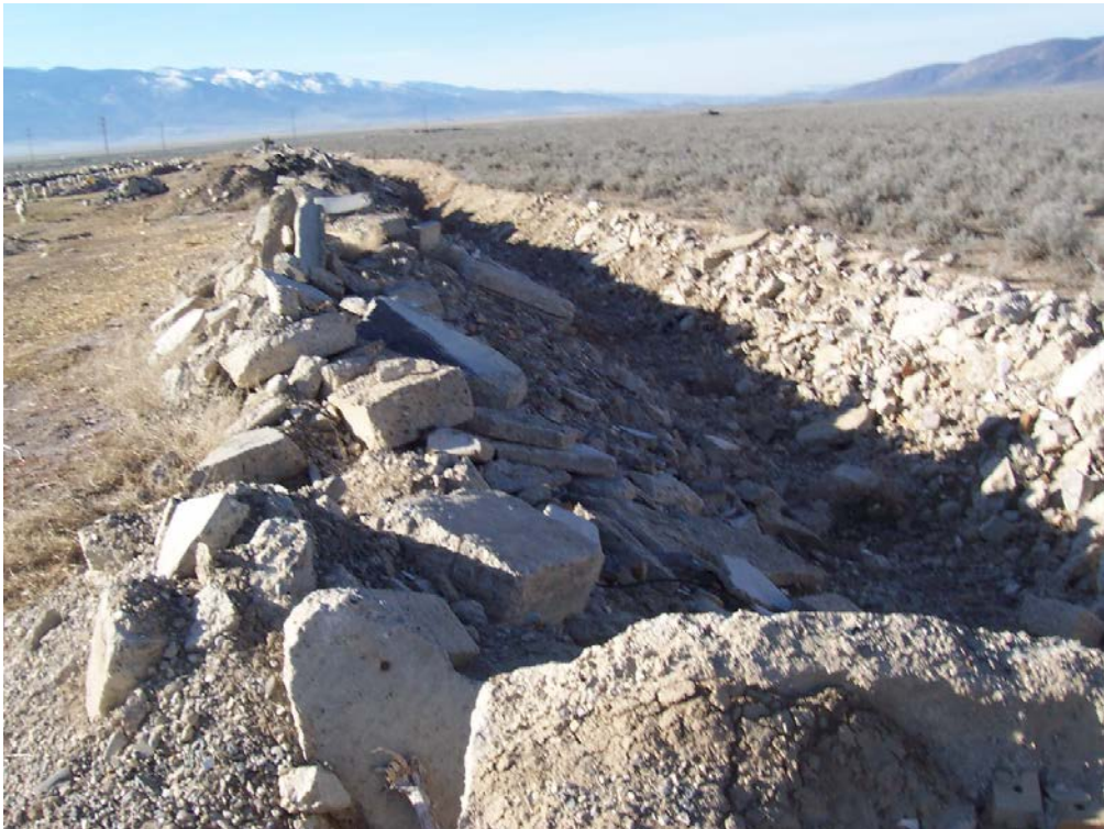
Channel with concrete placed as rip-rap
