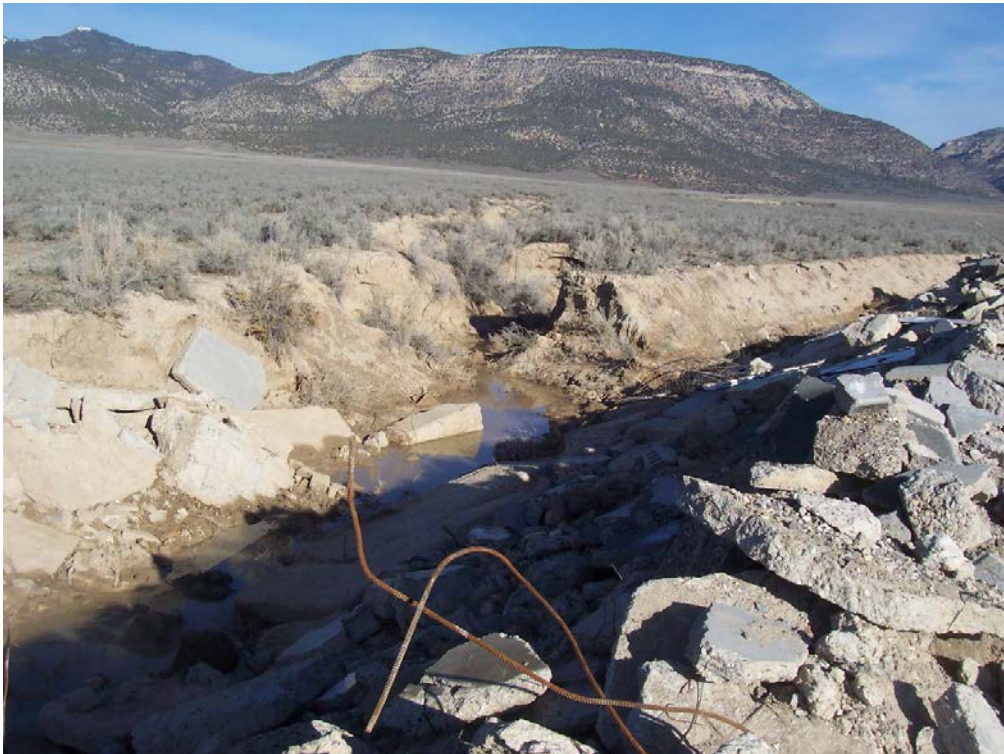
Rebuilt channel with concrete debris
