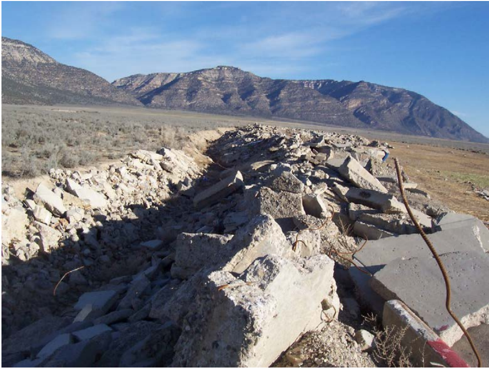
Channel with concrete placed as rip-rap
