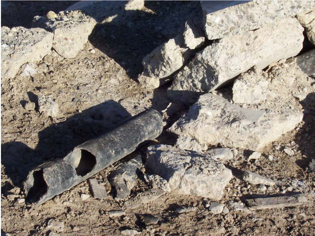
Waste cast iron pipe within the concrete debris
