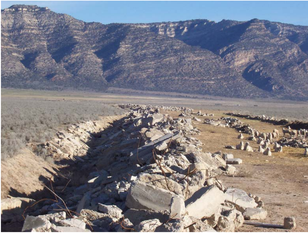
Concrete debris with channel
